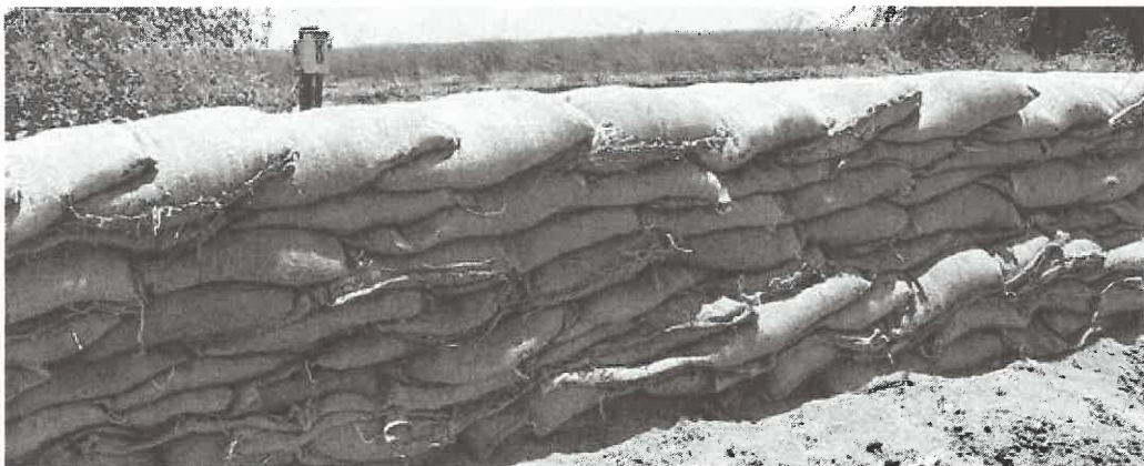
Sandbag Wall Construction
