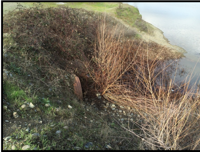
Figure 9. Site 9 - Existing Culvert Crossing
