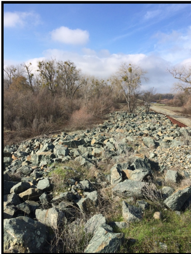
Figure 7. Site 5 - Existing Sheet Pile Wall – Feather River Side, Existing Rock Armoring
