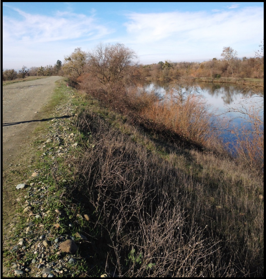
Figure 2. Site 2 - Inlet Weir Location Looking Downstream along the Feather River Levee
