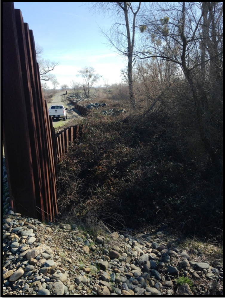
Figure 5. Site 5 - Existing Sheet Pile Wall – Feather River Side
